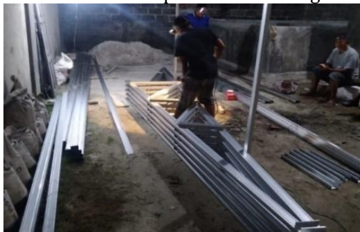
Figure 6 Assembling the Foundation and Roof of Angkringan
