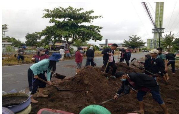
Figure 5 Soil Leveling at Angkringan Locations
