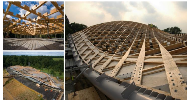
Gambar2. Rangka atap Savill Building
