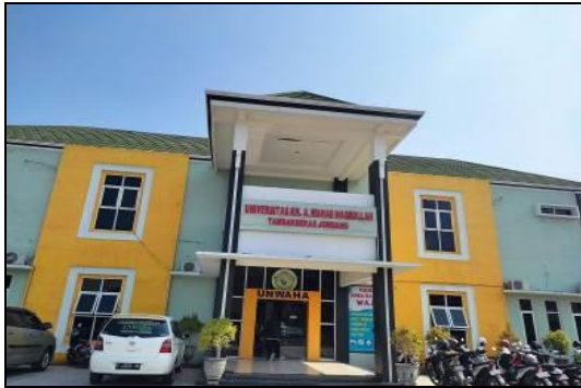
Picture 6 Office information sign
