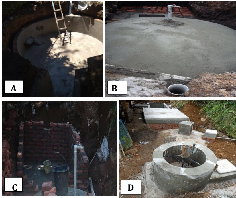
Figure 4. (A) Digester Casting; (B) Methane Gas Reservoir Installed by Faucet; (C) Making Cow Final Manure Shelter; (D) Communal Biogas with Final Disposal Sites
