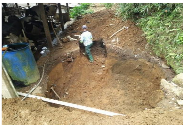
Figure 2. The digging process of the digester
