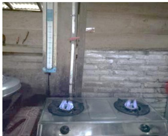
Figure 5. The stove with biogas from cow dung
